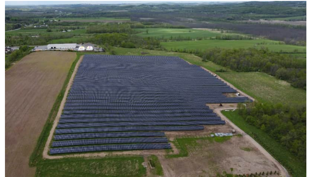
Community Solar Project Example
