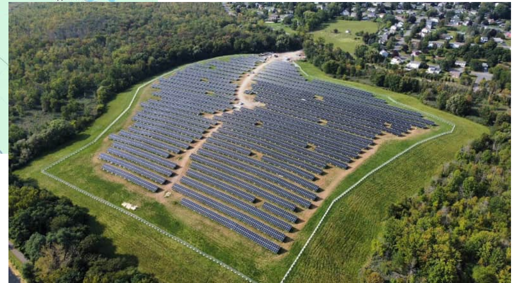
Community Solar Project Example
