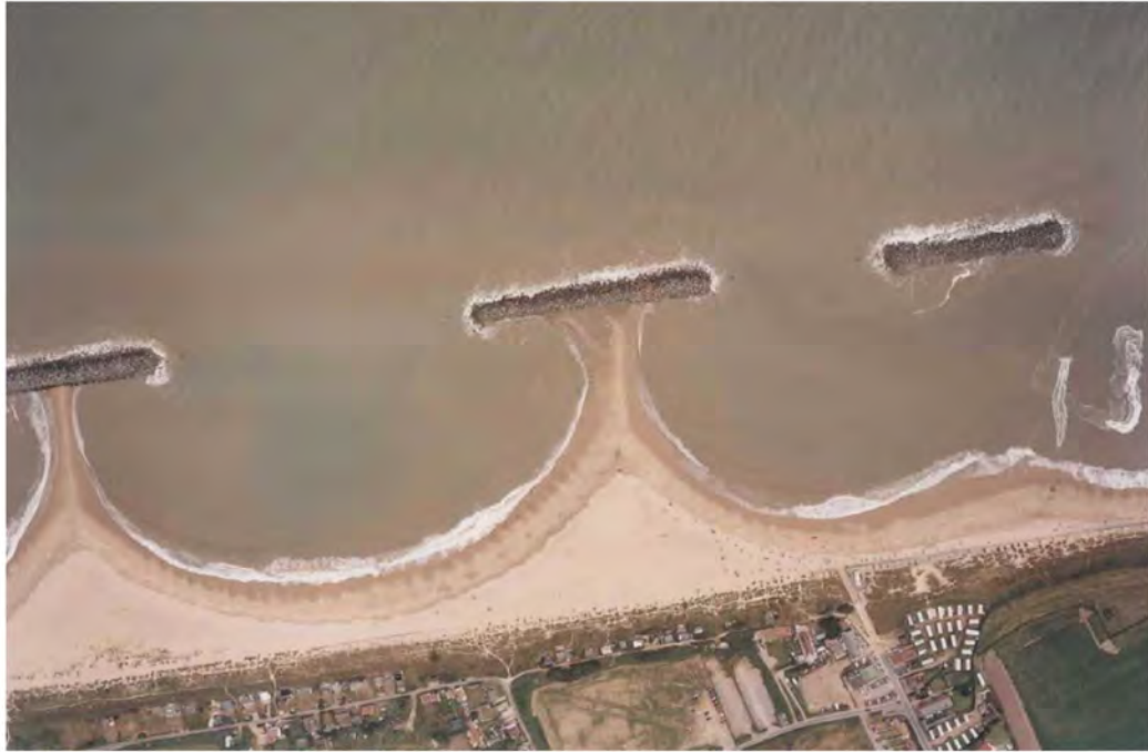
8: Example of tombolos and a salient and tombolos created behind detached breakwaters at Sea Palling, north-east Norfolk (2002). Photograph copyright Environment Agency.
