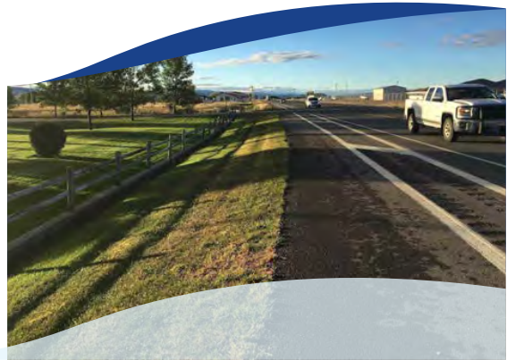
Figure 29: A buffered rumble strip zone creates a more comfortable paved shoulder. (Photo credit: Small Town and Rural Design Guide)
