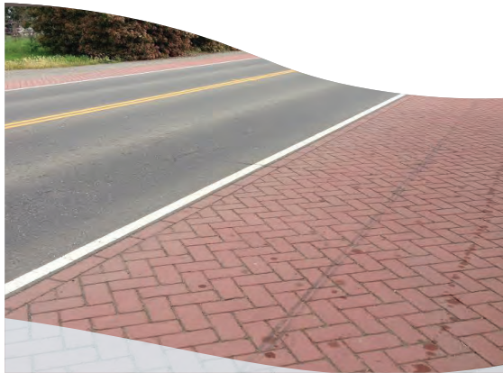
Figure 28: Pigmented, stamped asphalt mimicking bricks is used as emphasis on a paved shoulder. (Photo Credit: Small Town and Rural Design Guide).
