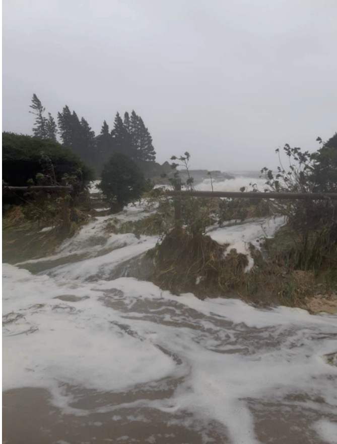
Dune blowout. Paths made in the sand dunes, allow for channels of water to spew onto the adjacent road.
