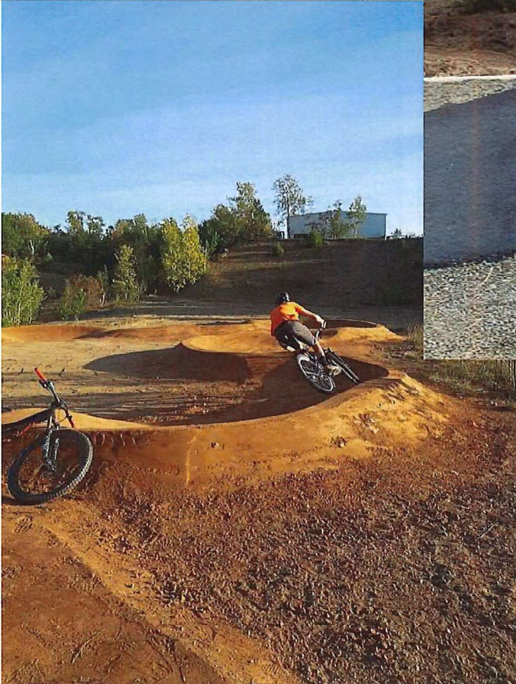
Pump Tracks with rollers and bermed turns. Surface can be soil, pavement, concrete or wood.
