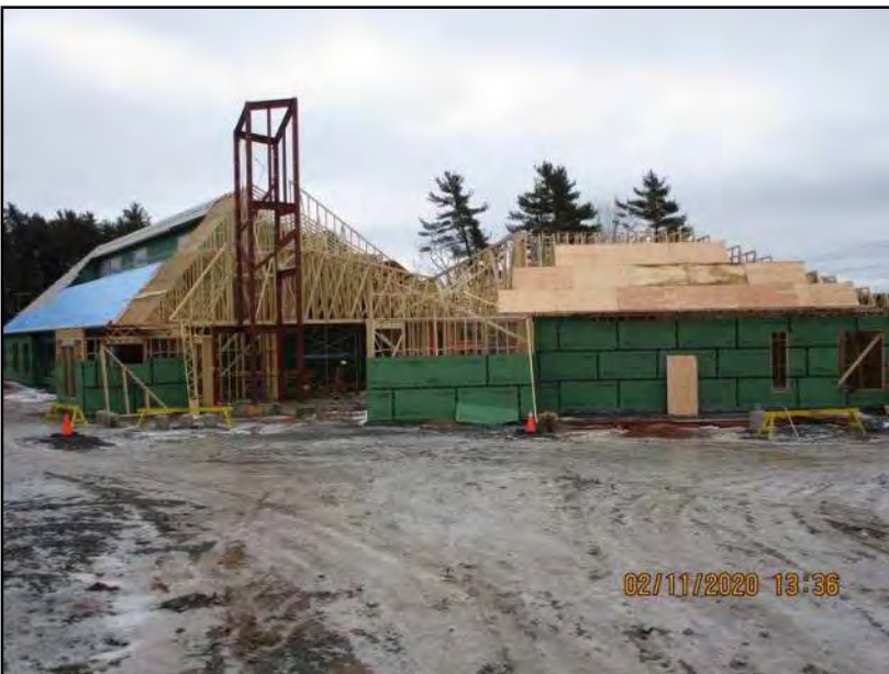
Pic 03 - Phase 3 roof sheathing commenced
