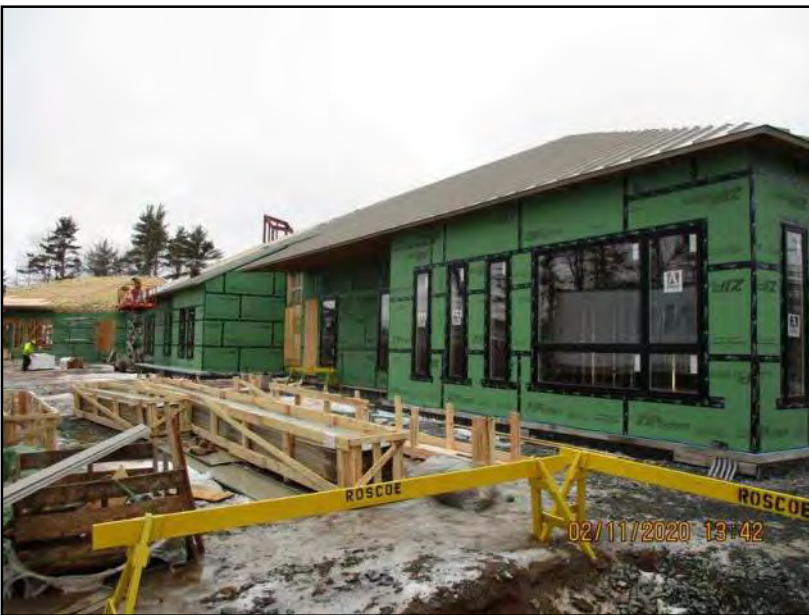
Pic 17 - South East corner
