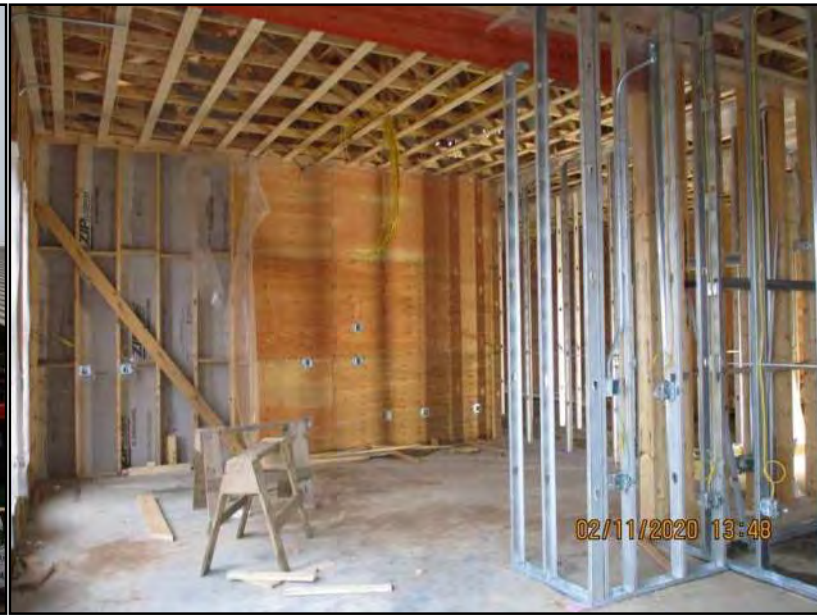
Pic 27 - Staff Room - electrical rough in
