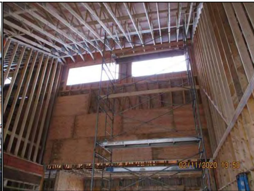
Pic 39 - WorkStations Rm: sheathing ongoing
