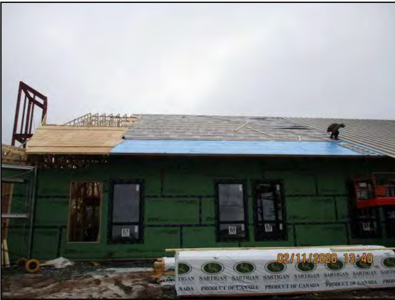
Pic 12 - Phase 2 Roofing: extent of underlay and blueskin
