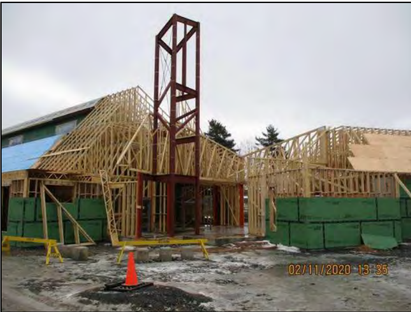
Pic 01 - Main entrance and exterior Bench piers
