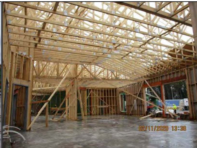
Pic 09 - Phase 3 roof trusses
