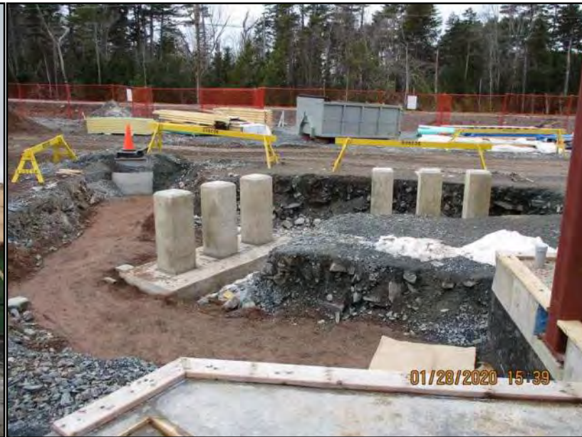
Pic 76 dated Jan 28th - Benches: Concrete piers
