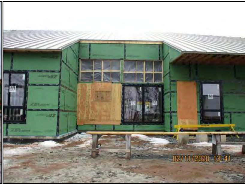
Pic 14 - South elevation at side entrance
