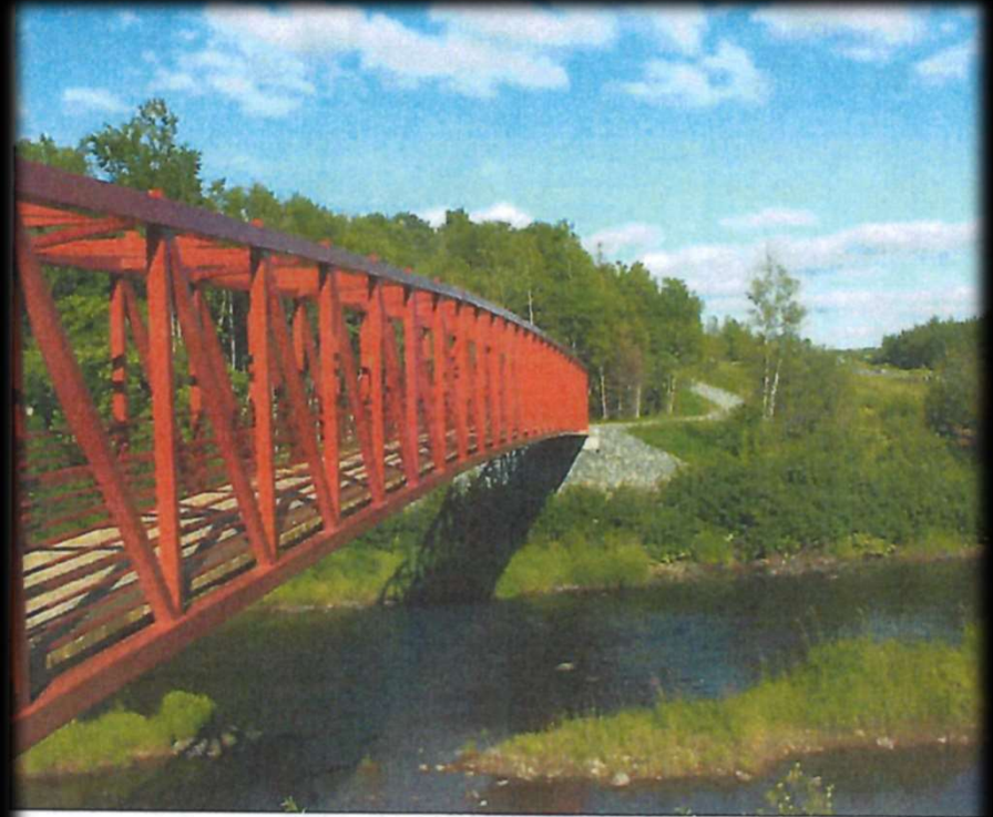
A photo of the River Philip Bridge located near Oxford, Nova Scotia
