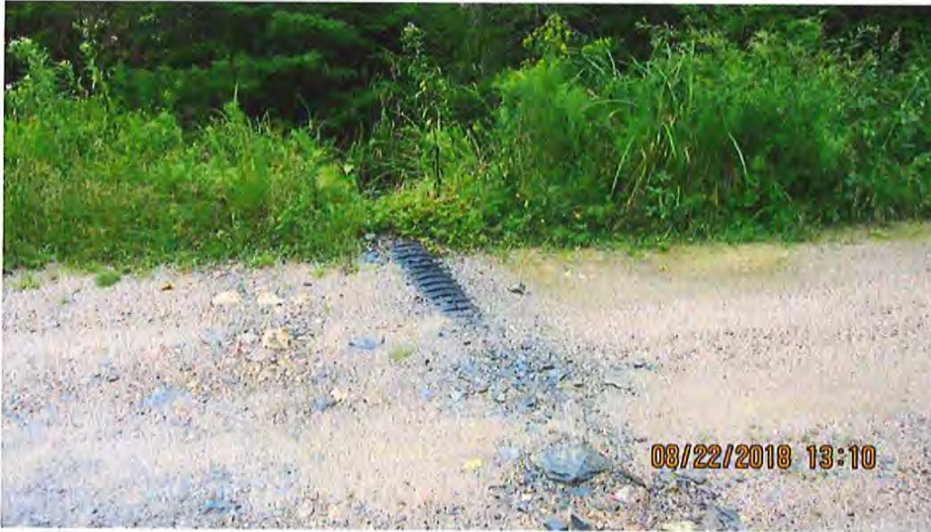
Woodstock Road exposed culvert. (Source: EDM)
