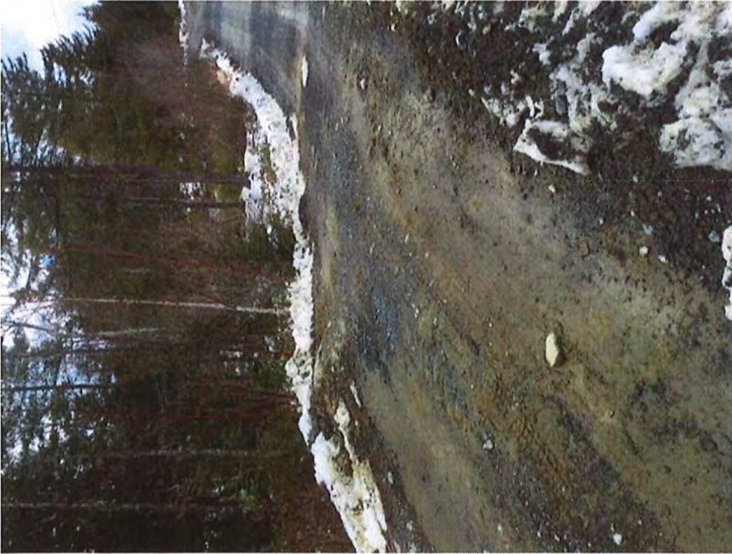
This last one doesn't do justice to the issue. You can see the huge rock the road was built over. The road is worn down, the dirt get soft and this is the spot that the fire truck cannot crest as it bottoms out.
