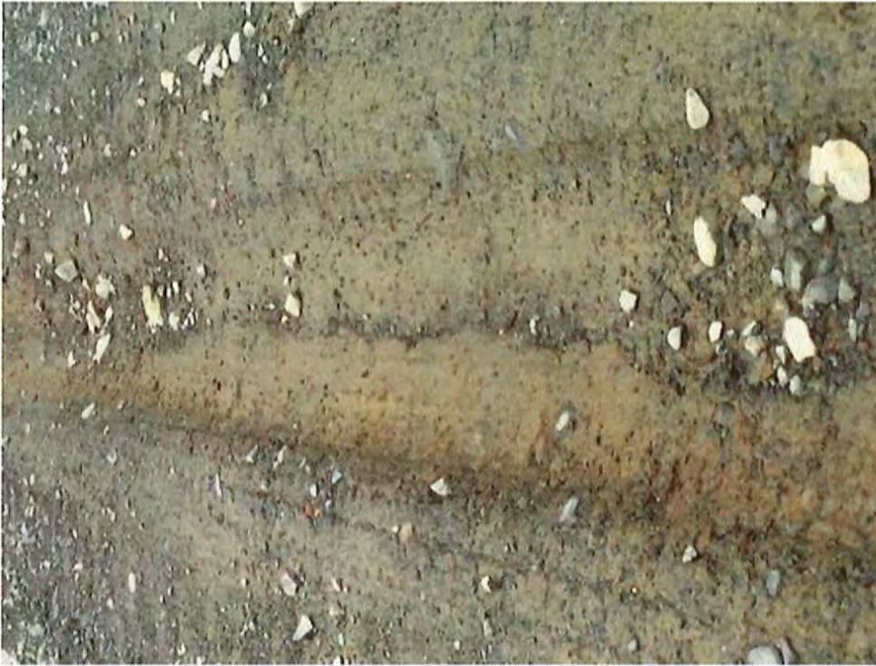
This last one doesn't do justice to the issue. You can see the huge rock the road was built over. The road is worn down, the dirt get soft and this is the spot that the fire truck cannot crest as it bottoms out.
