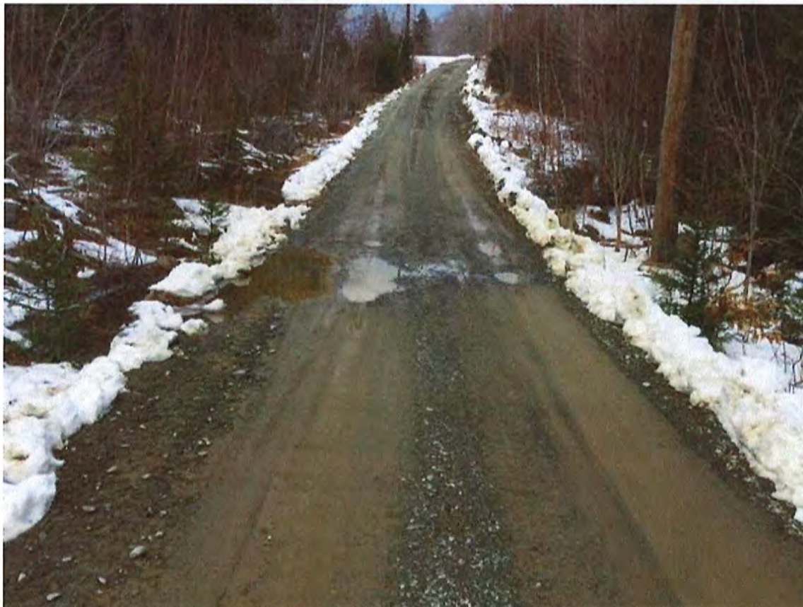
These two show no ditch and water drains across the road
