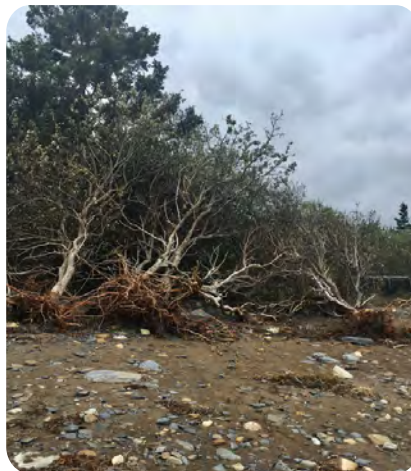
Coastal shoreline showing erosion, fallen trees, and debris along the water's edge, illustrating impacts to coastal property and natural areas.
