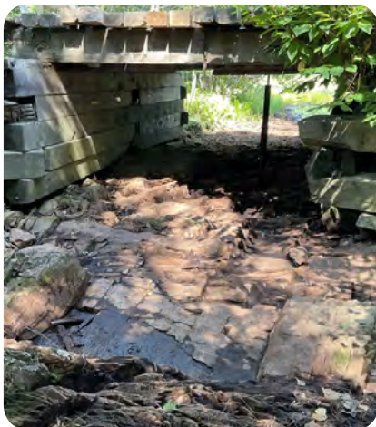
Dry streambed or watercourse beneath a bridge, showing low water conditions associated with drought.
