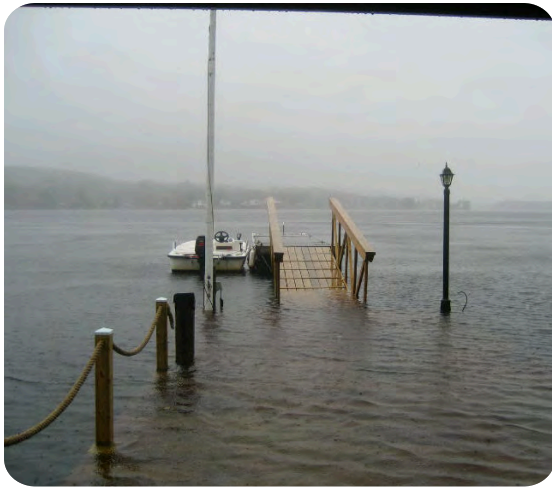
High water levels around a dock and shoreline infrastructure, illustrating flooding or storm surge conditions.
