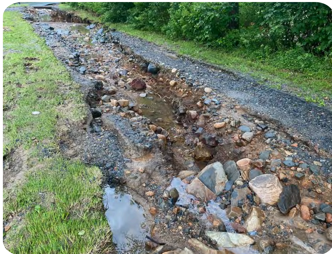
Washed-out roadway or driveway showing exposed rocks and erosion following heavy rainfall or flooding.
