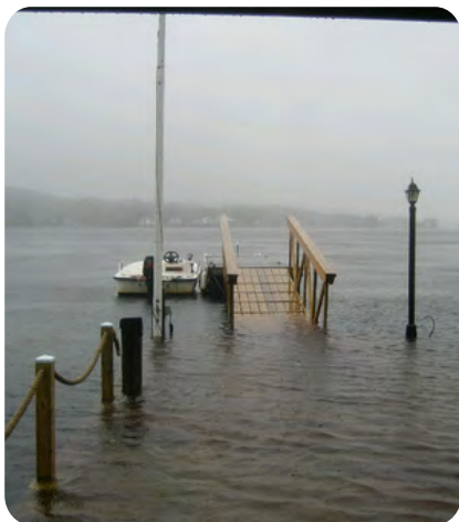
High water levels around a dock and shoreline infrastructure, illustrating flooding or storm surge conditions.
