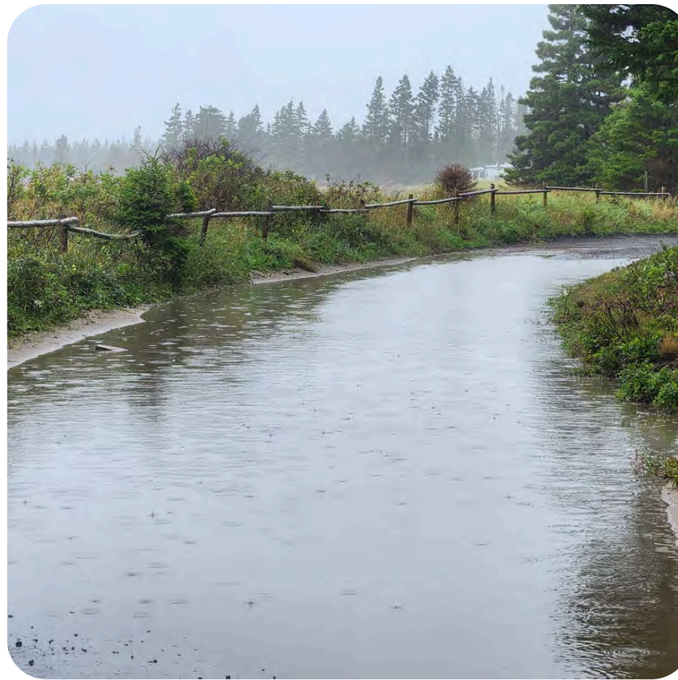
Roadway flooding after heavy rainfall, with water covering the road surface and restricting access.
