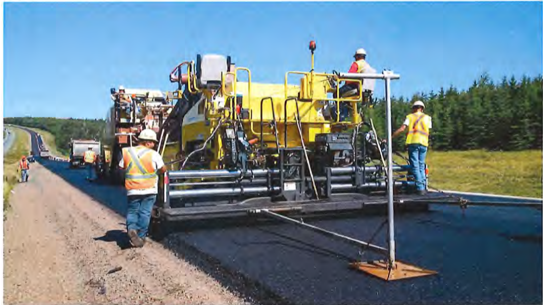
A repaving operation on Highway 104 in Cumberland County, near Amherst.
