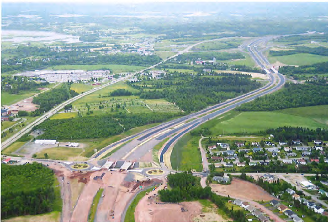
Highway 104 twinning, outside of Antigonish, showing construction of the Trunk 7 interchange, including a roundabout. (Photo courtesy of Ken Wright)
