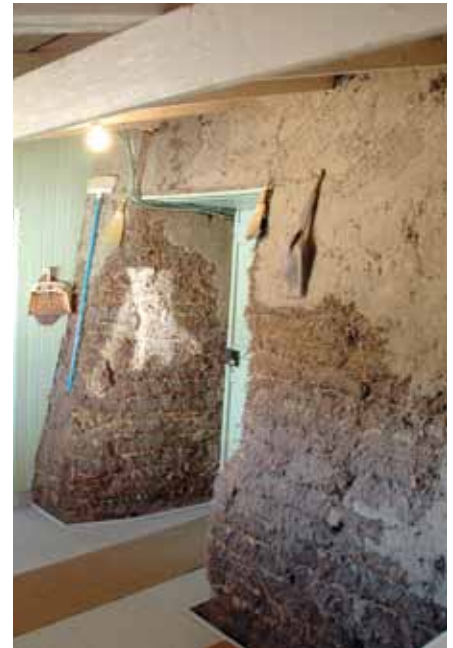
The lean-to is a character-defining element that shows the evolution of the Addison Sod House in Saskatchewan from a rustic sod dwelling to a comfortable home. Removing the later changes to restore the house to an earlier period would not be appropriate because it would remove elements that have heritage value.
