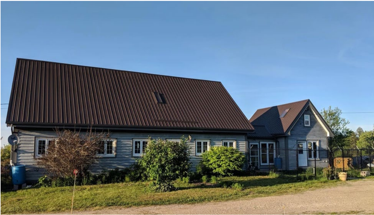
Figure 3. Example of the proposed metal roof style, constructed by Wall's Metal Roofing in Blockhouse, NS.
