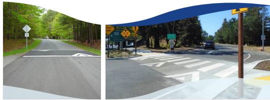
Figure 24: Examples of Traffic Calming. L: Speed table on a Rural Road, R: Raised crosswalk (Photo credit: Small Town and Rural Design Guide)
