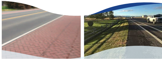
Figure 28: Pigmented, stamped asphalt mimicking bricks is used as emphasis on a paved shoulder. (Photo Credit: Small Town and Rural Design Guide).
